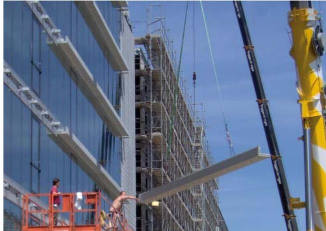
Fig. 1: CFRP prestressed HPSCC facade beams with L-cross section 267 x 385 mm and length 8.38 m
