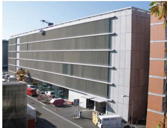
Fig. 2 CFRP prestressed HPSCC L-beams as structural facade elements
